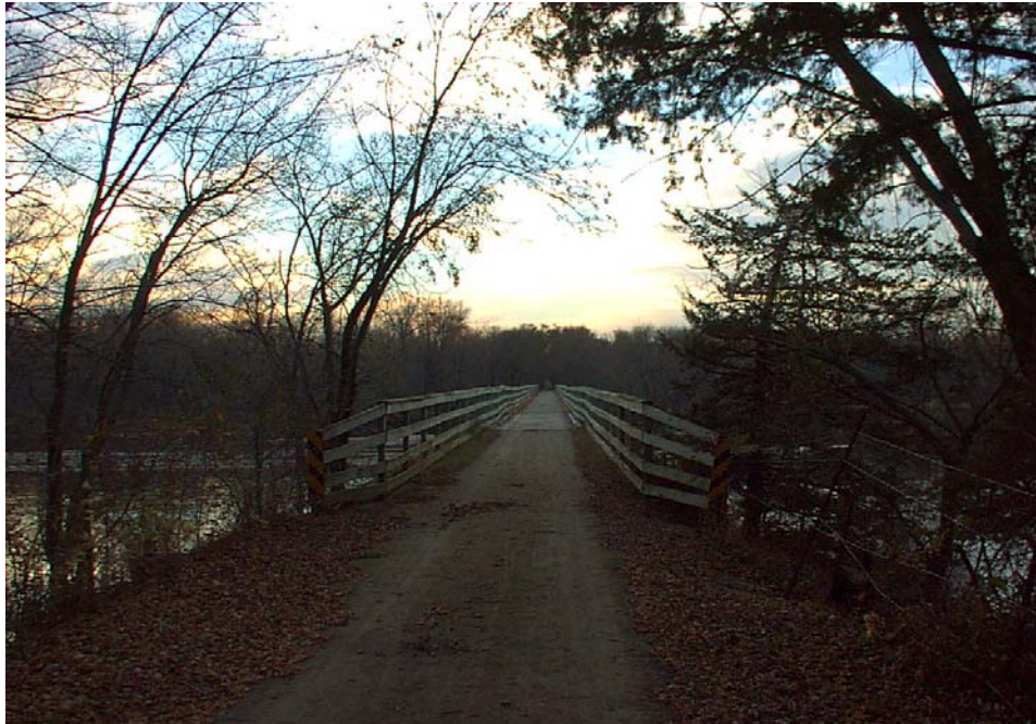
Bridge over the Cedar River on the Cedar Valley Nature Trail
